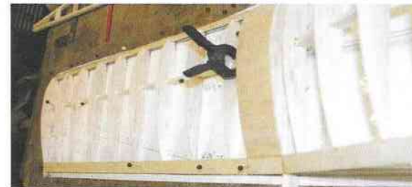
...the second panel is then built, propping up the first panel.
